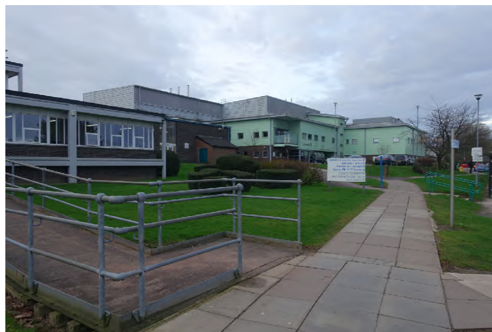
4. Pedestrian Route to Entrance 6
